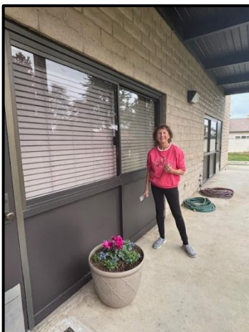
AFTER picture of the Voight Hall Panels
